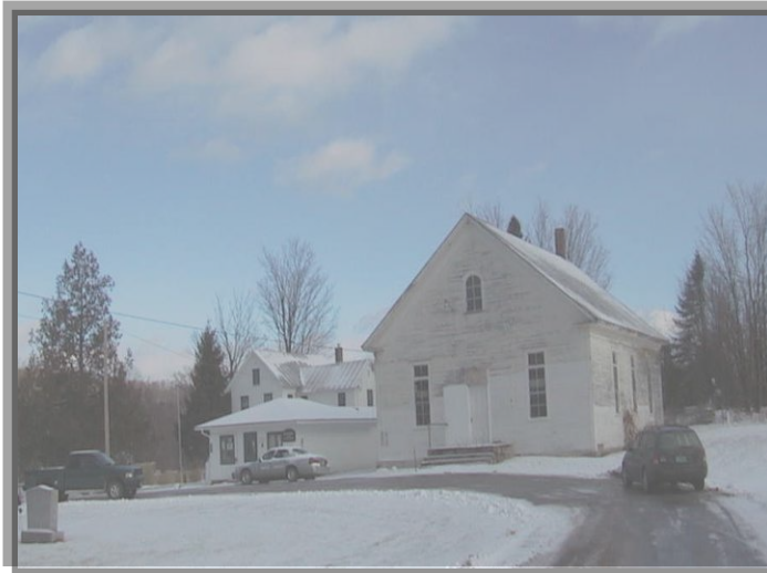
Berkshire Town Hall Before Renovations
